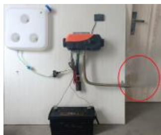
Excessive pump oil produces white smoke
